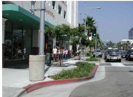
CORNER CURB EXTENSIONS extend the curb and pedestrian ramp further into the roadway and allow greater visibility for crossing pedestrians. As shown above, they create an opportunity for planting.
